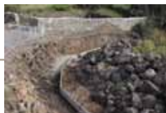
September 2016 - Flood defences.
