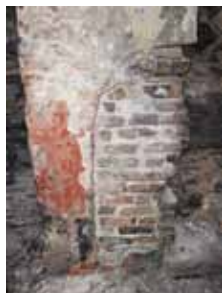
Arched fireplace (infilled), The East Cottage.
