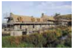
15 October 2015 - Roof to Cottages & House.
