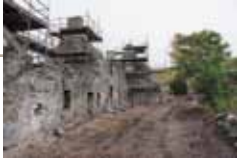
25 August 2015 - Repairs to the Georgian House.
