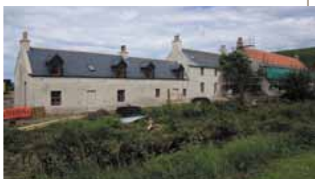
21 June 2016 - External works nearing completion.
