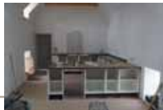
21 June 2016 - Kitchen installation underway.
