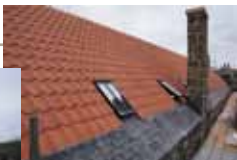
17 May 2016 - Pantiles and Scotch Slate on Sail Loft roof.
