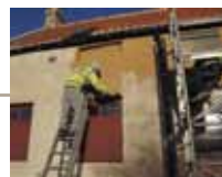
November 2016 - Application of Lime Wash.
