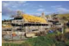
25 September 2015 - Roof structure on Cottages.
