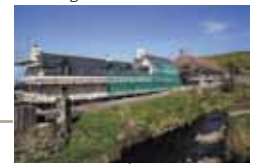
19 April 2016 - Harling complete on Cottages.
