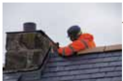
15 March 2016 - Lead work on chimney.
