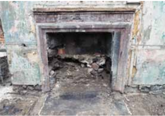
Wooden fire surround, Georgian house.
