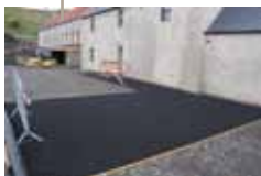
October 2016 - Car Park
