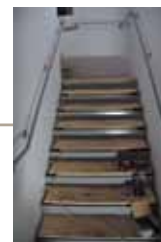
16 June 2016 - Staircase in Georgian House.
