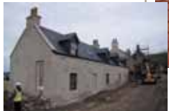
17 May 2016 - Scaffolding down.
