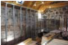
10 December 2015 - Inside the Cottages.
